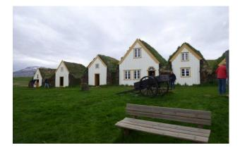
This complex set of turf buildings is a warren of rooms linked by a central passageway and a number of additional farm outbuildings. The conservation requirements are clearly very complicated with ongoing treatment of issues of damp, mould and degrading wall materials. All repair work is undertaken with the help of detailed recording and original material is retained where possible.
